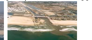
Fig 13. Resuspended Sediments as a Result of Dredging Activities.
